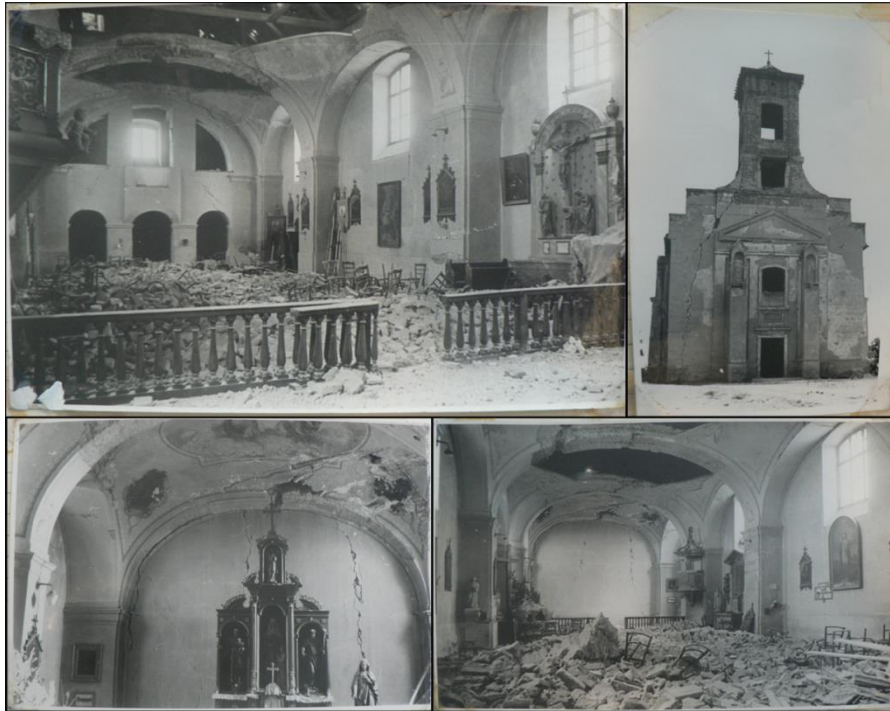
Fig. 1 The ruined Szent Anna parish church after the earthquake in Dunaharaszti, 12 th Jan. 1956 (Historia Domus 1956)
